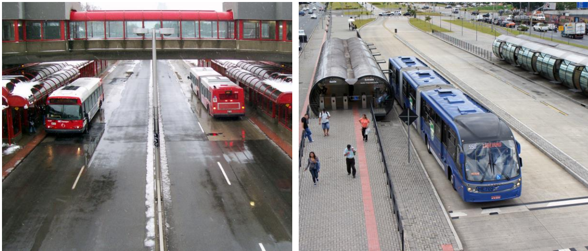
Figure 11: Ottawa (left) and Curitiba (right) BRT stations
