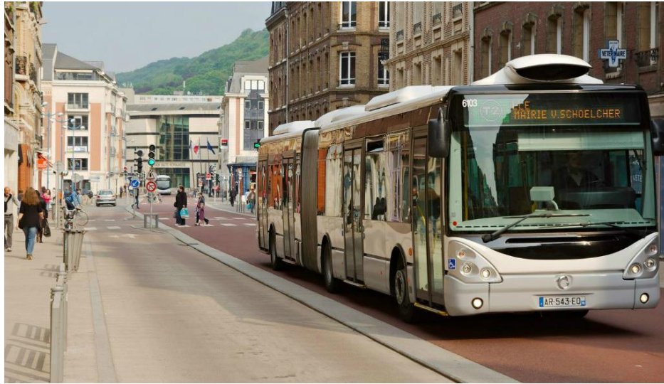
Figure 2 - Avenue Alsace-Lorraine: TEOR infrastructure in city centre
